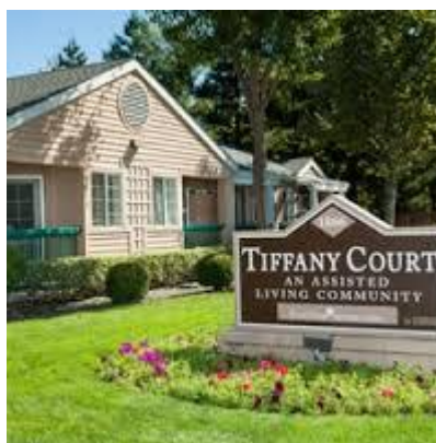
Figura 8 - Tiffany Court of Walnut Creek – Entrada Principal
